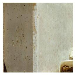
Above photo shows concrete column where Zemdrain® was used with conventional formwork on the right hand side leaving an uncontaminated, blowhole free surface and on the left no Zemdrain® was used resulting in a blowhole and blemished surface.
