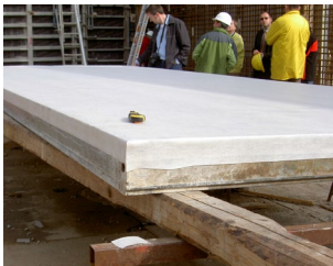
Zemdrain® MD self-adhesive fixed to the formwork
