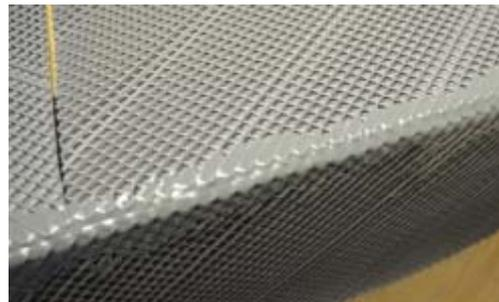
**2mm x 40mm seam of Polyurea WCS gun grade using large diameter static mixer (gunned similar style to a sealant) with manual gun. Excellent seam join between 2 adjoining strips of Proofex Engage.**
