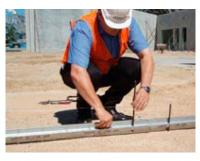
**Step 4.** Return to first stake, raising the metal Keyjoint to the height of the slab or string line, then twist stake 90° to lock the Keyjoint in place with pliers or spanner. Repeat this at the last hole and continue to drive the rest of the stakes in place.
