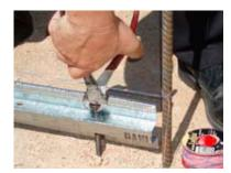
**Step 6.** Line up capping to edge of Keyjoint and press over top edge. Continue pressing capping firmly over the rest of the Keyjoint length.
