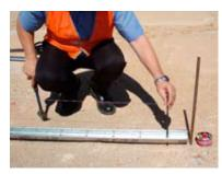
**Step 2.** Drive the first stake through small oblong hole near end of Keyjoint, ensuring the flat section of the stake is in line with the flat section of the hole. Place Keyjoint along string line and rest on the ground.
