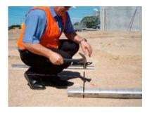
**Step 3.** Hammer stake 10 mm below height of Keyjoint in the first hole of Keyjoint length. Next repeat the same in the last hole in Keyjoint length (4 stakes per 3 m length are recommended).
