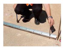
Step 1. Set up your work area by placing a string line along the joint line. Set string line at the height of the finished floor level. Lay out Keyjoint along this line. Please note: if you are using capping, please allow for this height when setting up string line.
