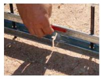
**Step 5.** Add joining clip if joining two or more Keyjoint lengths.
