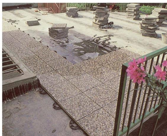
Helasto-ring can be set on multilayer bituminous waterproofing, on bituminous sheathing waterproofing or on synthetic sheet waterproofing.
