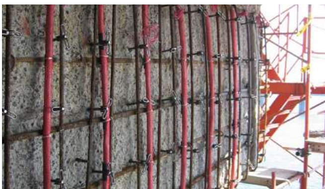
Galvanic anode system on bridge pier prior to concrete placement.
