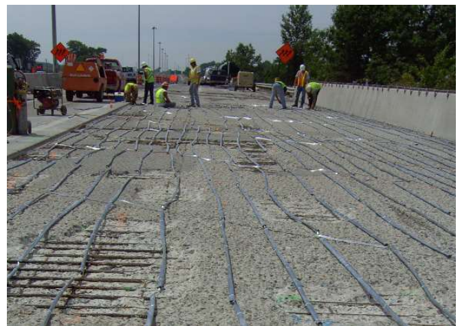
Galvanic anode system on bridge deck prior to placement of reinforced concrete overlay
