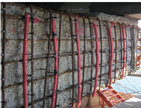
Galvanic anode system on bridge pier prior to concrete placement.
