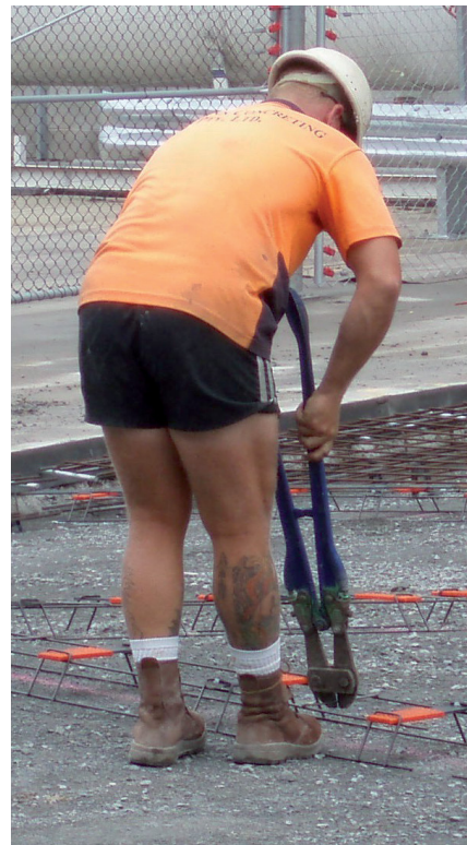
Cutting cross wires once cradle is correctly positioned.
