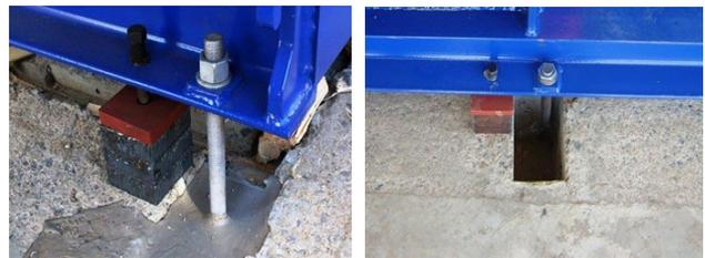
Typical levelling screw arrangement
