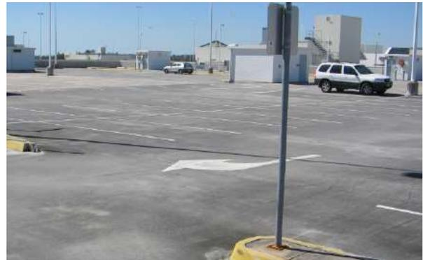
Rain damaged roof deck resurfaced with Aegis MSP
