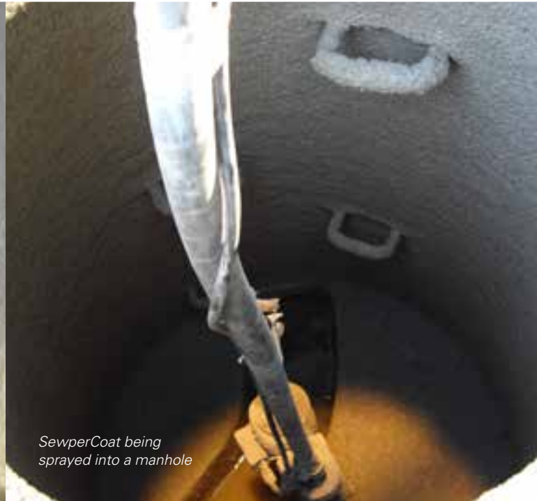
Spray application of Nitocote EP500 inside sewer
