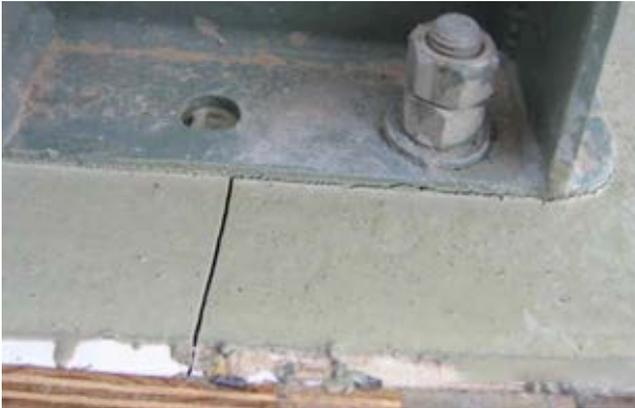
The image on the left shows a significant crack in an epoxy grout which was initially a concern. However, investigation revealed the crack was only in the perimeter grout and didn't extend under the baseplate. The crack was later sealed with a low viscosity epoxy mix to stop water infiltration and for appearance's sake.
